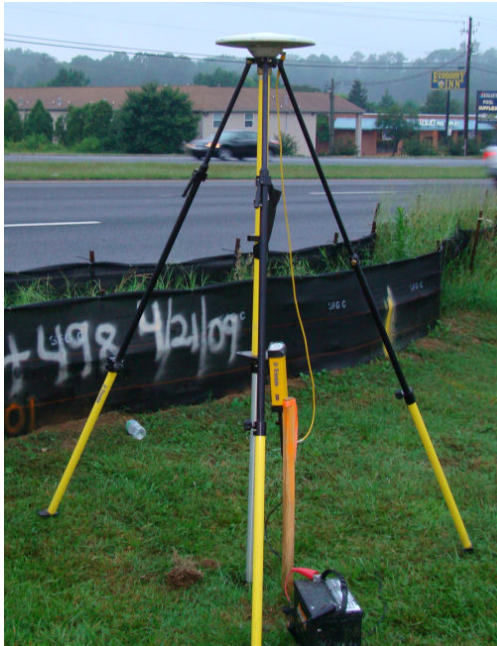
GPS Base Station
